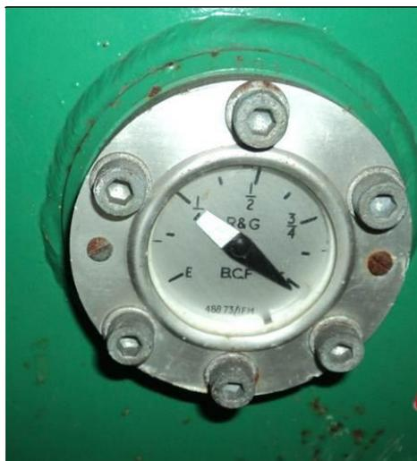
If the quantity of halon gas within a cylinder, extinguisher or system is not provided on a label or is not otherwise evident, then it is advised that you liaise with your halon system maintenance contractor. Service and Inspection Reports on Halon units are the most reliable source for obtaining accurate halon gas quantity data. The example below shows an extract from a Service and
